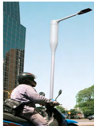
Micro cell on a lighting pole
